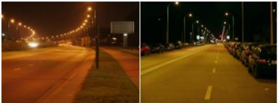
Figure 2: Geometrically structured, regular line of the points of light (optical arrangement) and high uniformity of illumination of the road determine the aesthetics of street lighting to the greatest extent.
