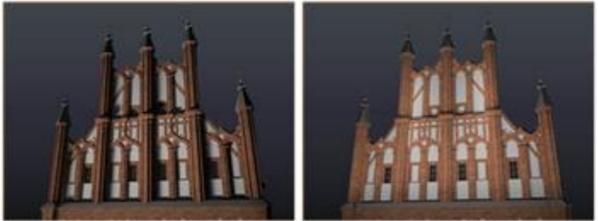
Figure 4: The illumination is considered as aesthetic in such projects, where both – light and shadow are used at equal level (on the left). The object which is fully illuminated frontally is considered as unesthetic (on the right).
