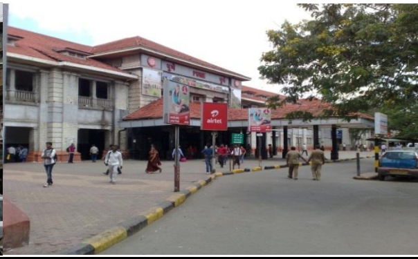
Pune Railway Station
