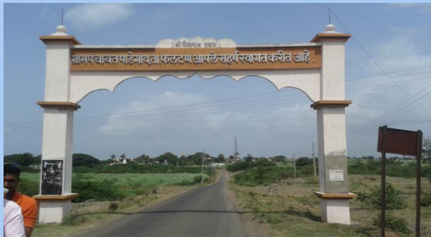
PHOTO 21: CONNECTED ROAD WITH
