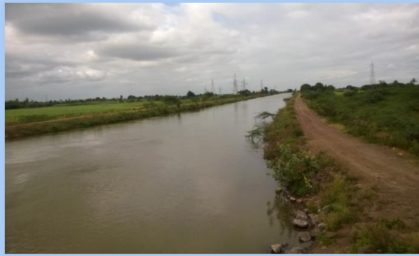
PHOTO 35: THE NIRA RIGHT BANK CANAL
