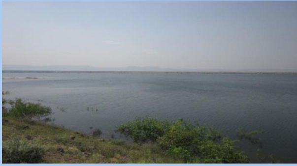
PHOTO 33: THE BANGANGA DAM
