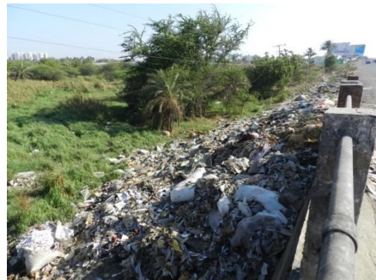
Photo 36: Sewage dumping in the stream
