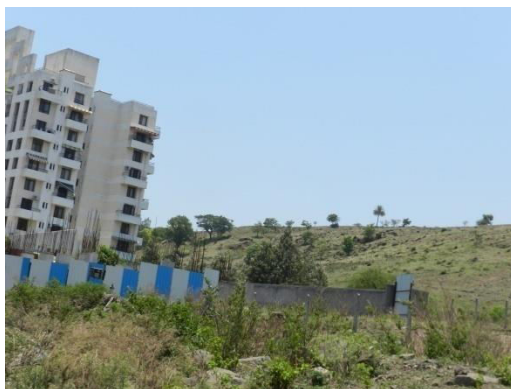
Photo 5: Construction on Hill Slope (Bavdhan Area)
