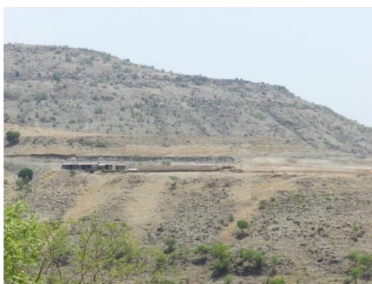
Photo 28: Hill cutting at upper catchment area
