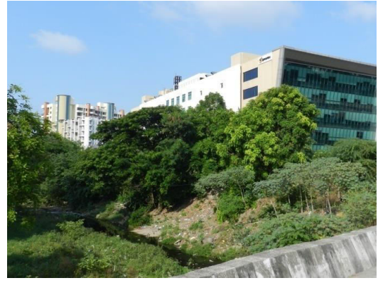
Photo 4: Construction and Dumping near Channel
