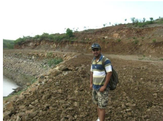
Photo 16: Slope cutting near Bhilarewadi Lake
