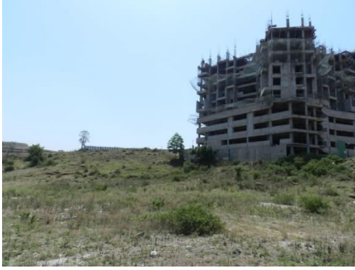
Photo 9: Construction on stream near Chandani chowk – Bawdhan
