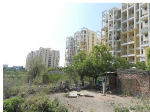
Photo 6: Construction on Stream (Banner - Pashan Road)
