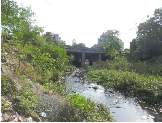
Photo 3: Dumping in Channel
