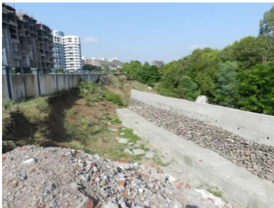
Photo 1: Retaining wall in Ram Nadi channel (Front View)
