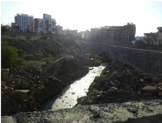
Photo 39: Stream blocking by construction in Kharadi
