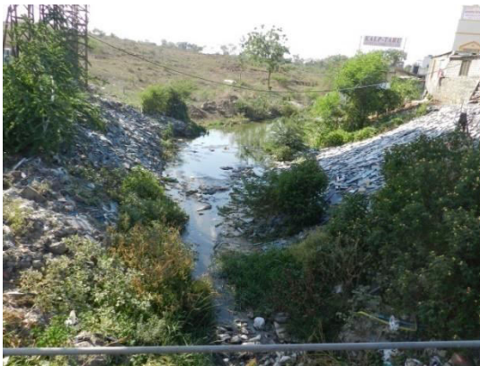
Photo 35: Construction material in the channel at Nagar road highway
