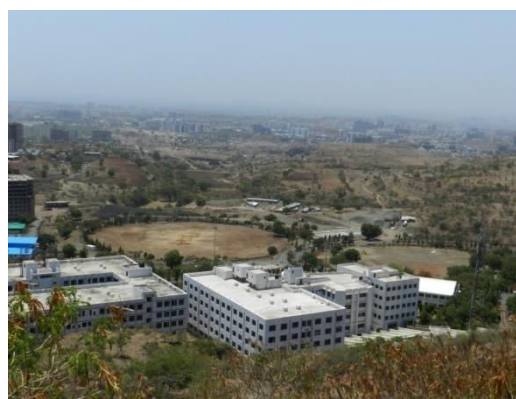
Photo 29: Construction at hill slope
