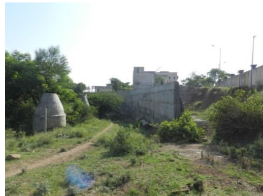
Photo 2: Retaining wall in Ram Nadi channel (Back View)
