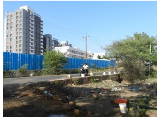
Photo 38: Construction of school on stream (Stream blocking)
