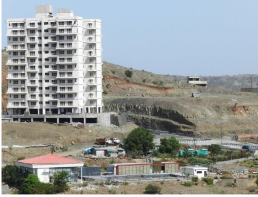
Photo 24: Hill Cutting at Kondhwa road
