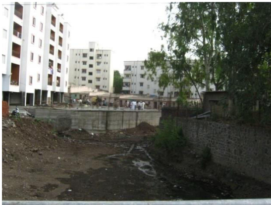
Photo 15: Construction in Channel at Mangadewadi
