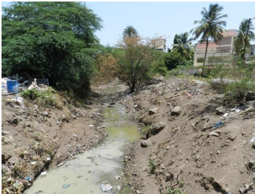
Photo 26: Construction material along the channel
