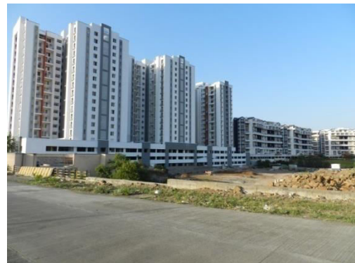
Photo 40: Construction on Stream
