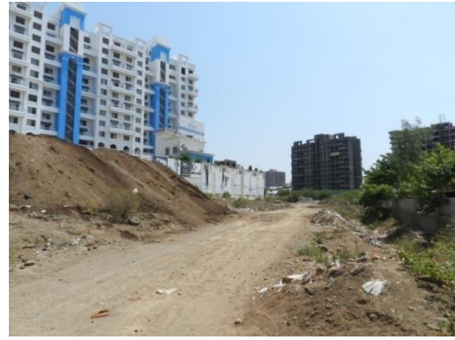
Photo 31: Construction and dumping along the stream
