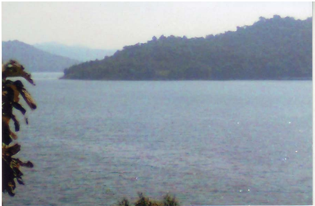
Inside view water level at Hetawane Dam
