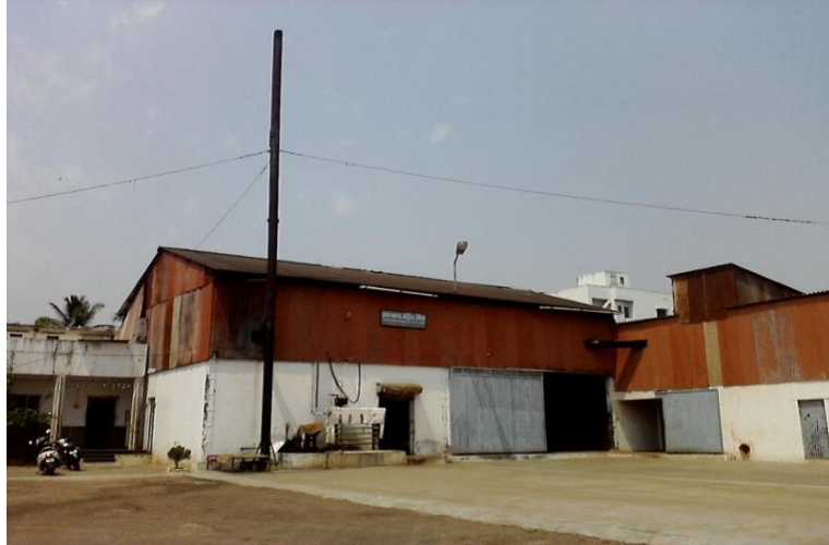
Photo Plate No.23: Exterior view of Groundnut oil mill. (M/S Jai Bharat oil near shahu market yard, Kolhapur, Tal: Karveer.)
