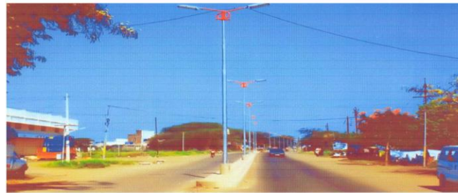
CFL- STREET LIGHT
