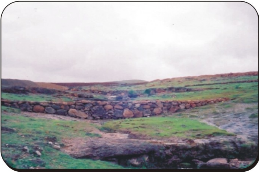
Loose boulder structure
