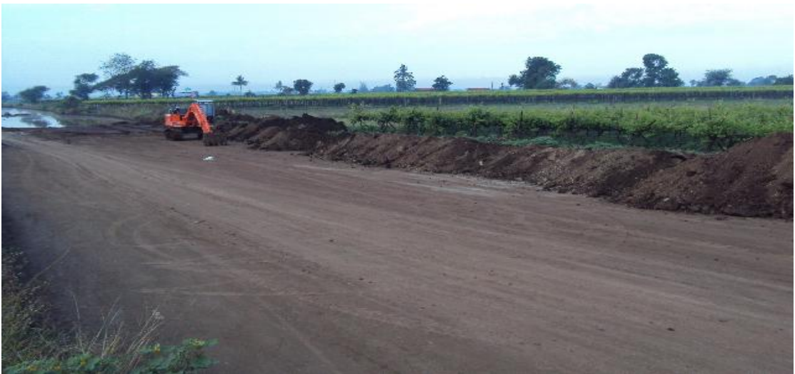
Photo plate no.29: Construction of New roads or bypass
