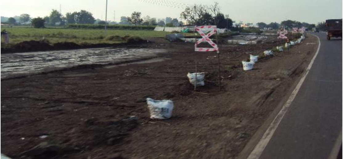
Photo plate no.28: Increasing the width of National High-way
