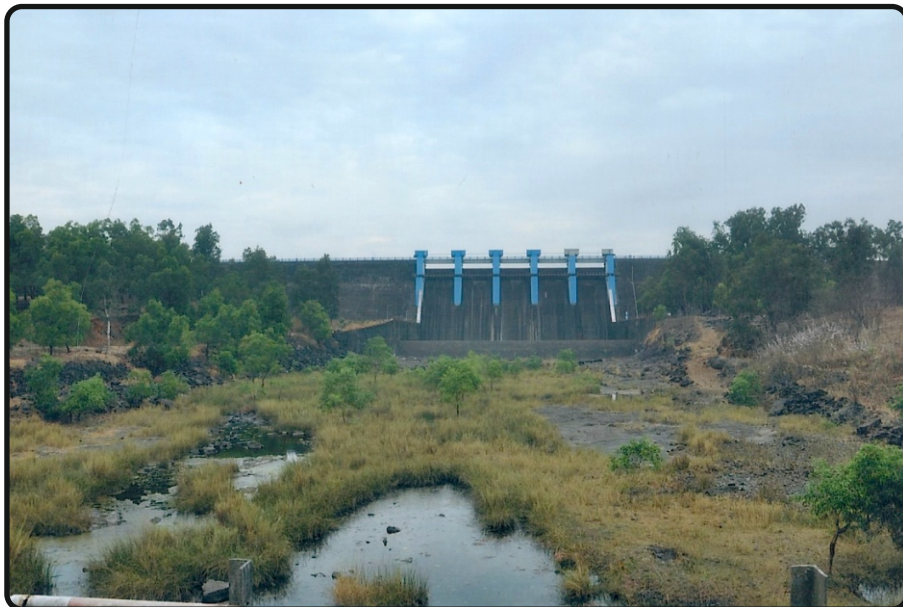
Vaitarna Dam North Gate
