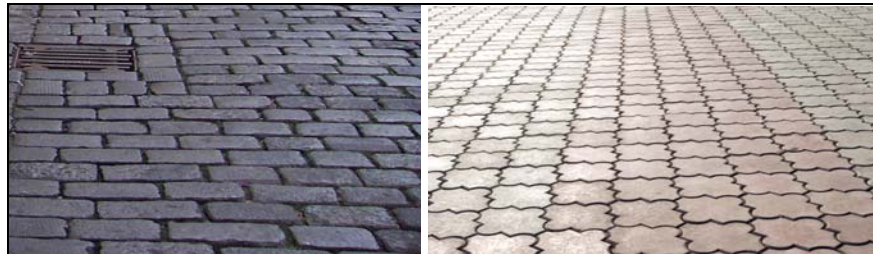
Photo 5.2 Pavers blocks street road & footpath
