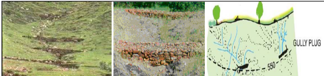
Figure 3.21 Gully Plug Technique
