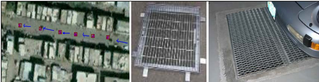
Figure 5.6 Recharge Pit along Road
