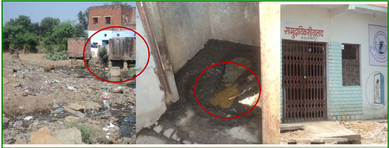
Photo: 7.3 Existing Status of some Toilets along with Modern Bio-toilet
