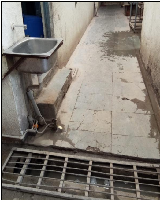
Pipeline Likage and missmanagment of water supply system
