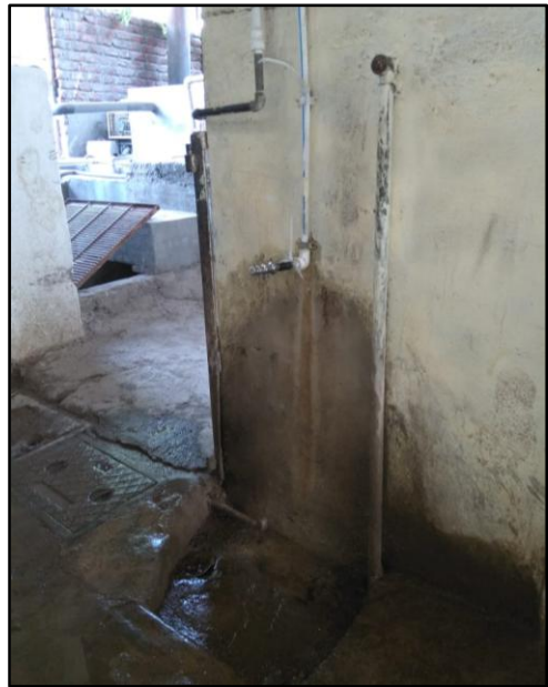
Pipeline Likage and missmanagment of water supply system
