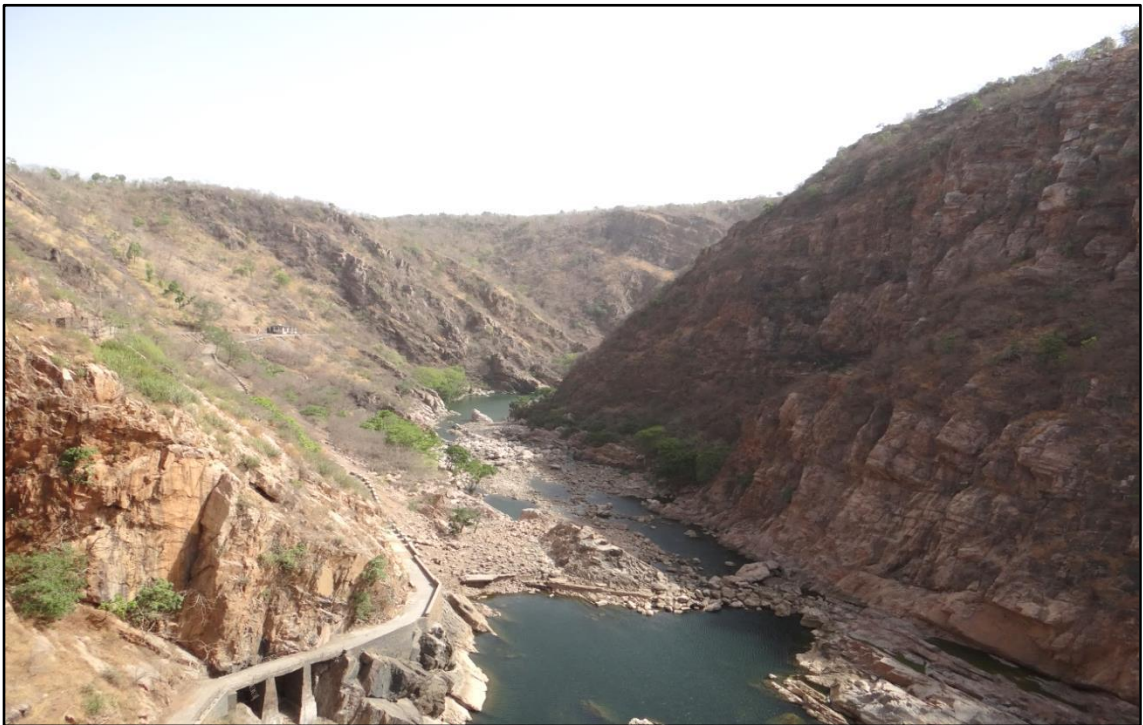
Figure 4.15: A view of deep and narrow gorge of the Jakham River downstream of Jakham Dam (Pratapgarh, Rajasthan)
