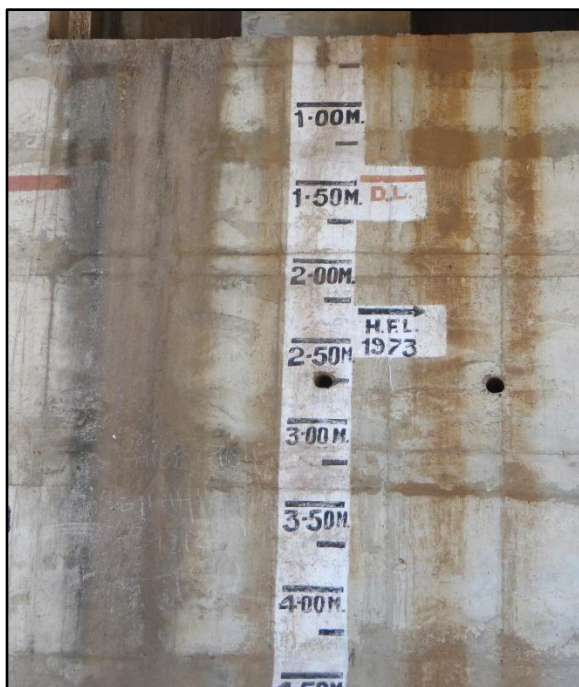
Figure 4.41: HFL mark of 1973 flood on the Mahi River on railway bridge near Timba Road railway station (Godhra, Gujarat)
