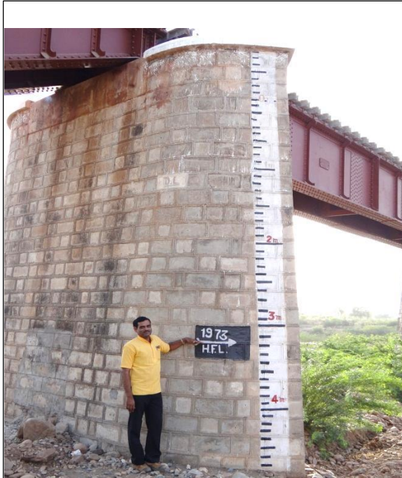
Figure 4.44: HFL mark of 1973 flood on the Som River Railway bridge near Depur (Dungarpur, Rajasthan)
