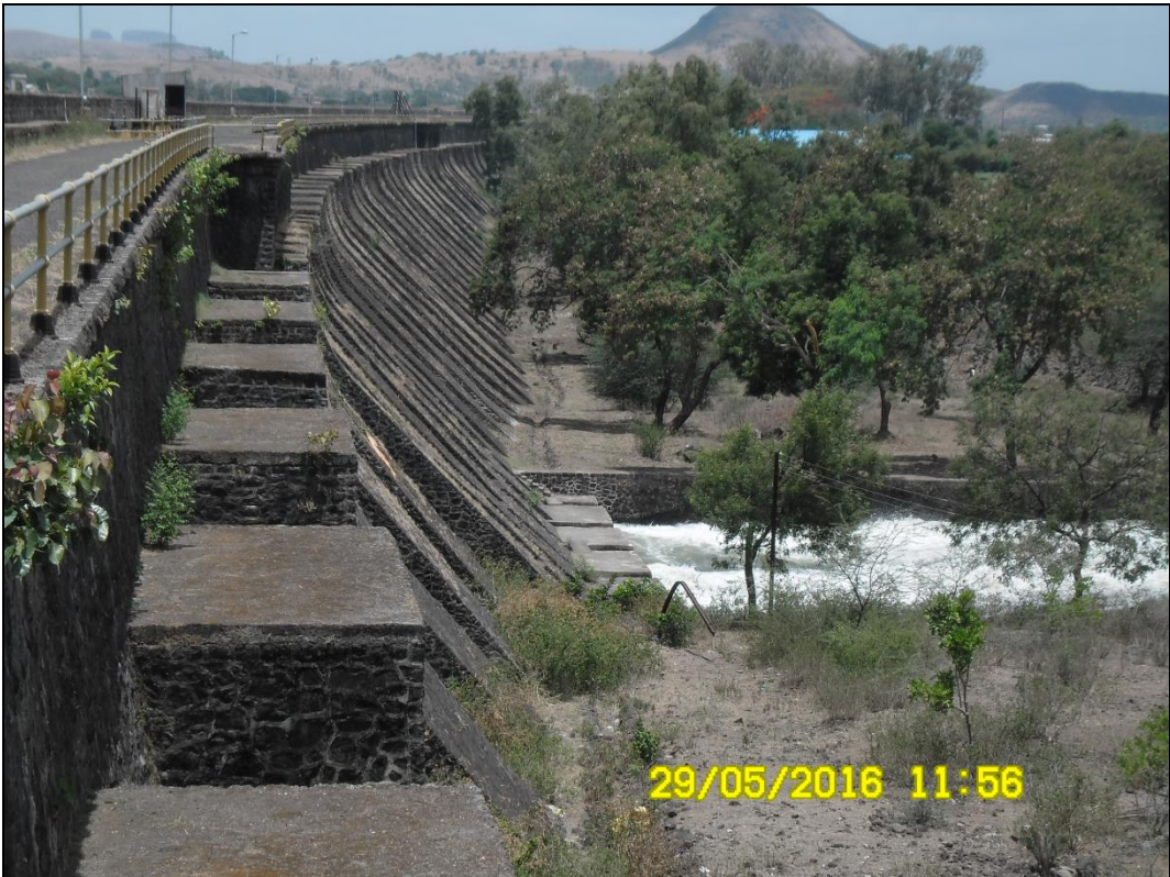
Photo 14: Darna Lake Reservoir Wall
