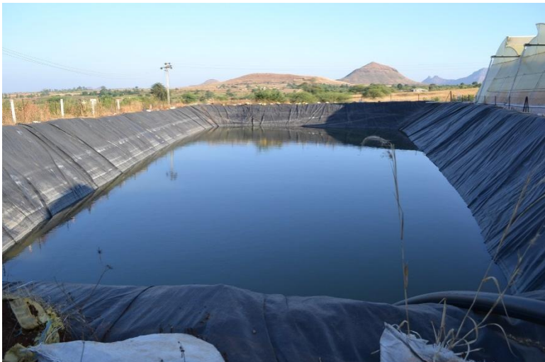
Photo 24 Fish Water Tank
