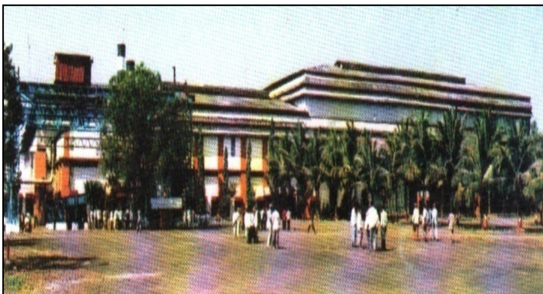
Photo No. 3: Gadhinglaj Factory Building
