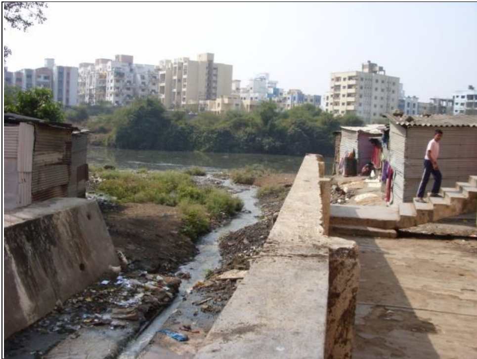
(a) Dirty water drainage in Pawana Nagar slum
