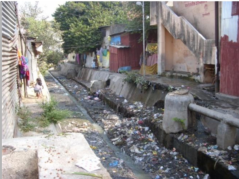
(b) Toilet seat near dirty water gutter in Gawali Nagar slum
