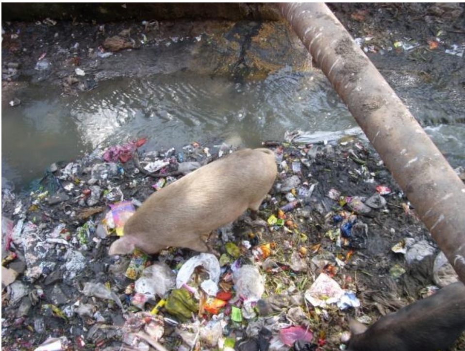
(b) Water pipe line passing through in gutter
