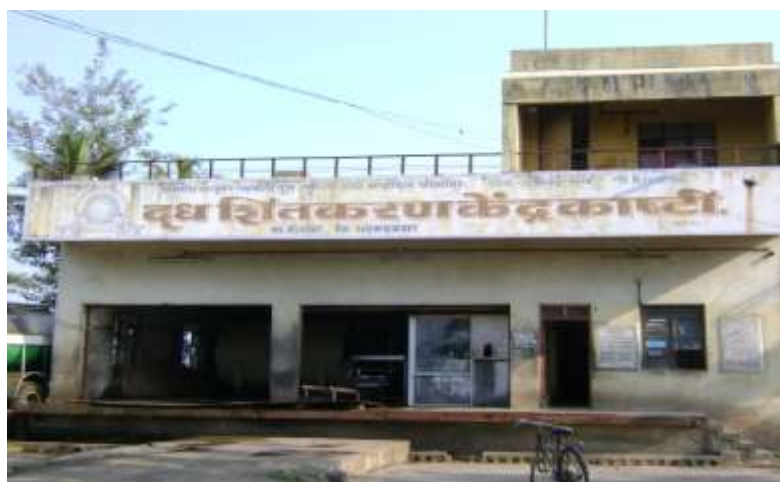
[Photograph No.44 Co-operative Milk Chilling Plant at Kasti]
