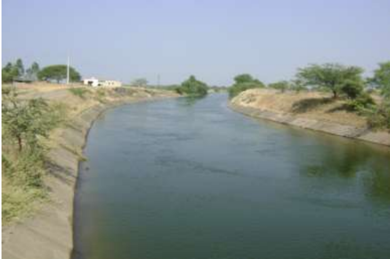
[Photograph No.4 Visapur Dam Joint Canal]
