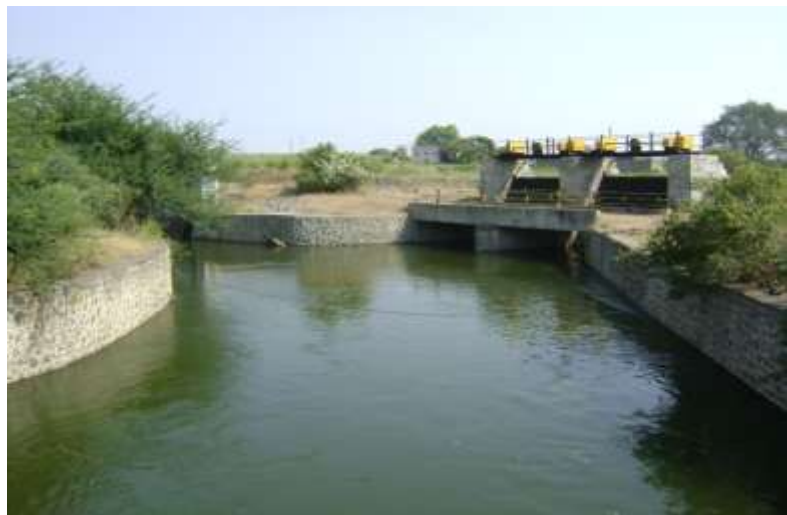
[Photograph No.14 Kukadi Project-Visapur distributory Canal]
