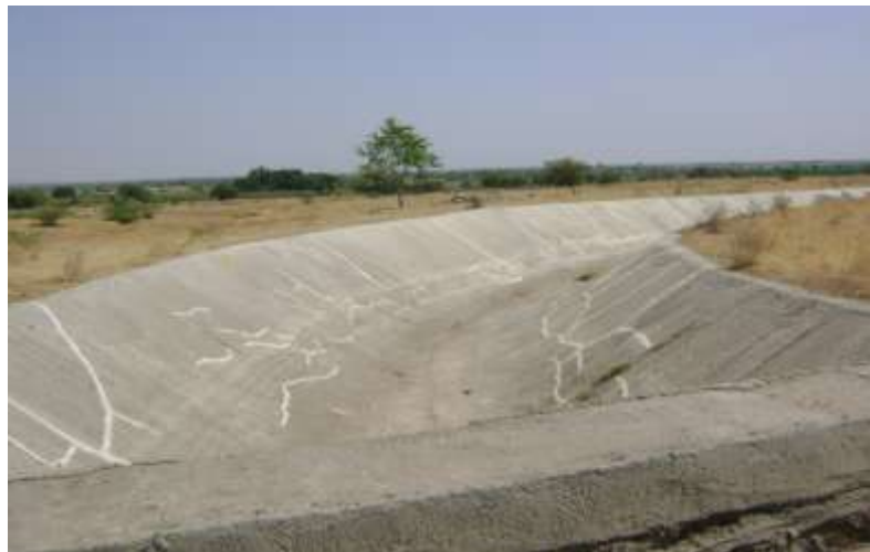
[Photograph No.8 Concrete Water Canal Kukadi Project]
