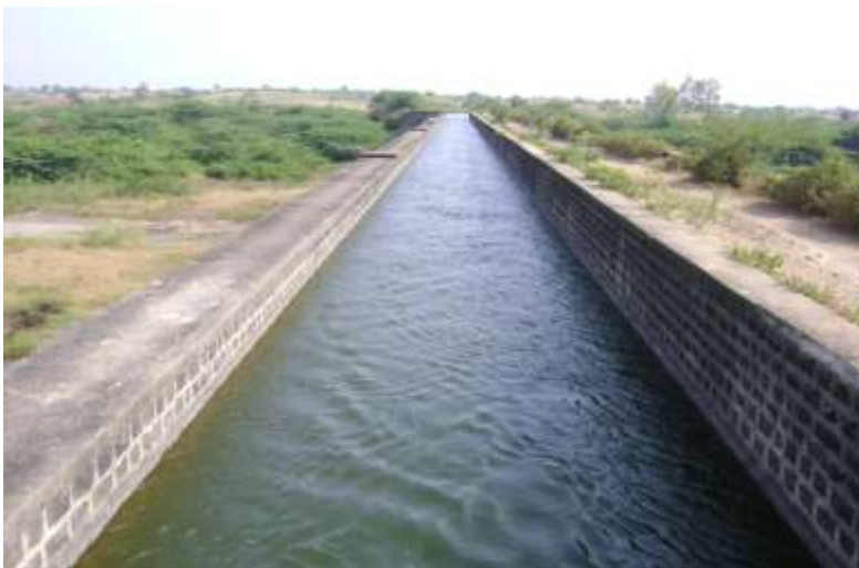
[Photograph No.3 Visapur Canal- Built by British Government]
