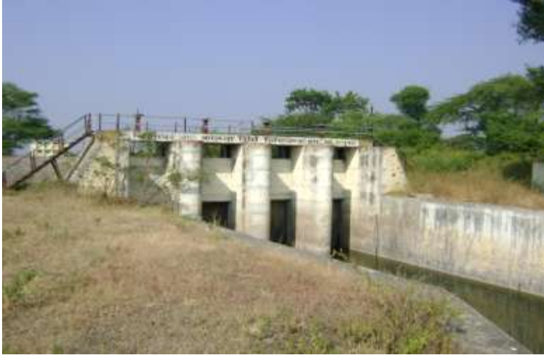
[Photograph No.13 Visapur Sub Canal No. 0/210]
