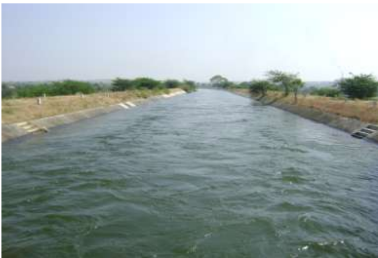
[Photograph No.6 Ghod Dam- Left Bank Canal]
