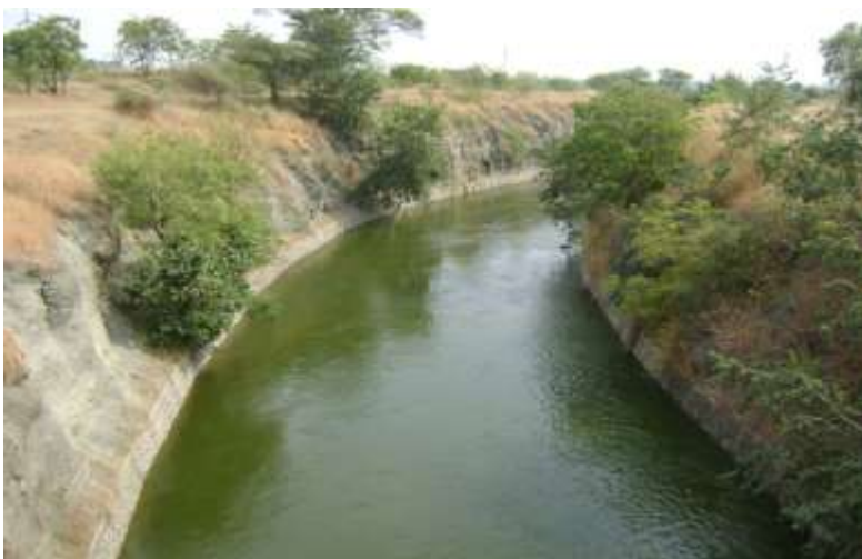
[Photograph No.9 Main Left Bank Canal- Kukadi Project]
