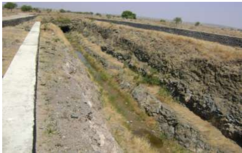
[Photograph No.11 Water Tunnel- Bhose Khind, Length 14 Km.]
