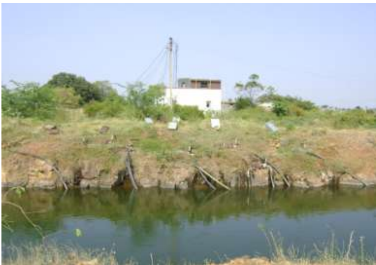
[Photograph No.12 Water Lifting from Ghod Left Bank Canal]
