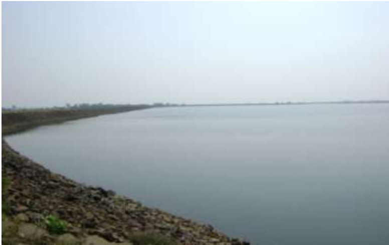
[Photograph No.1 Visapur Dam near Visapur]
