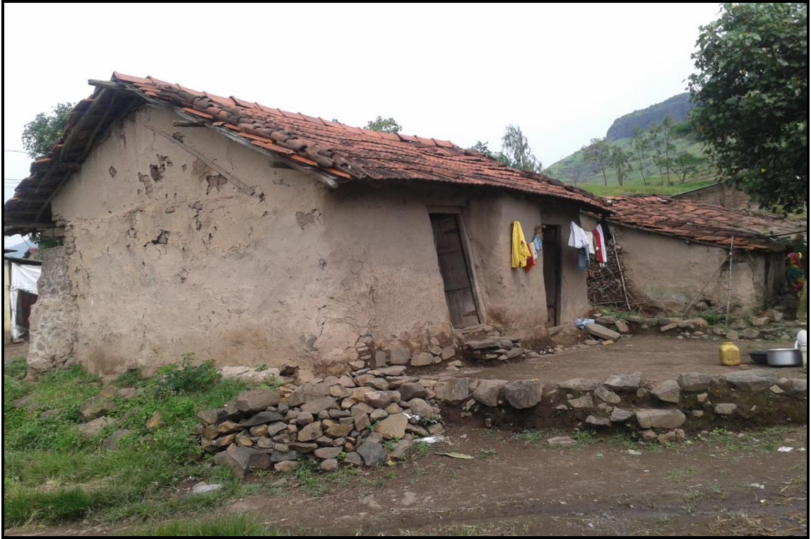
Photo-13: Typical Tribal House (Mud and Stone) at Ramshej Village in Dindori Tahsil.
