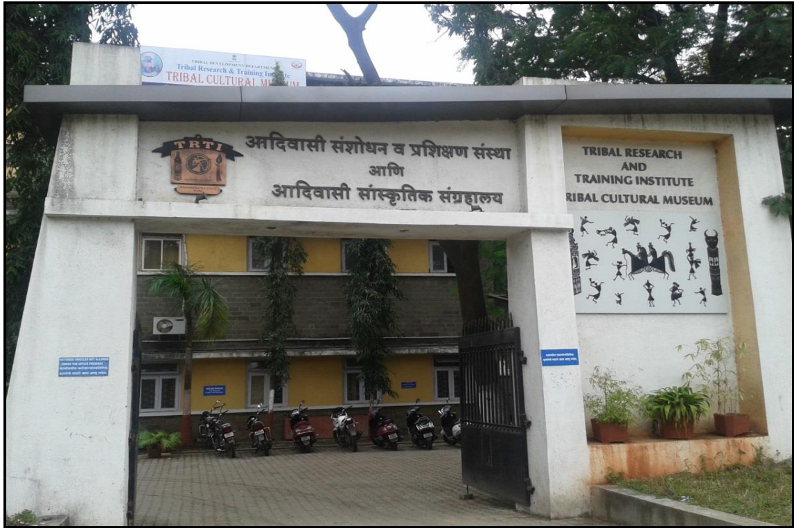
Photo-3: Building of Tribal Research and Training Institute at Pune.
