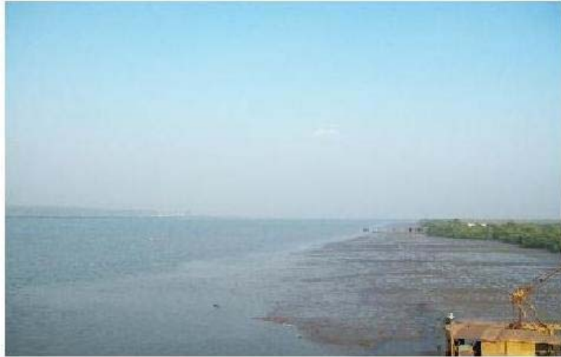
PHOTO PLATE: 1 VIEW OF KUNDALIKA CREEK FROM REVDANDA BRIDGE
